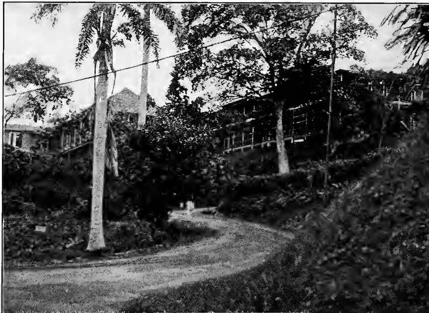
A BIT OF ANCON HOSPITAL GROUNDS
